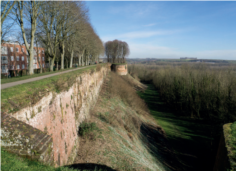
Three kilometres to walk on top of the wall and another three around the base
