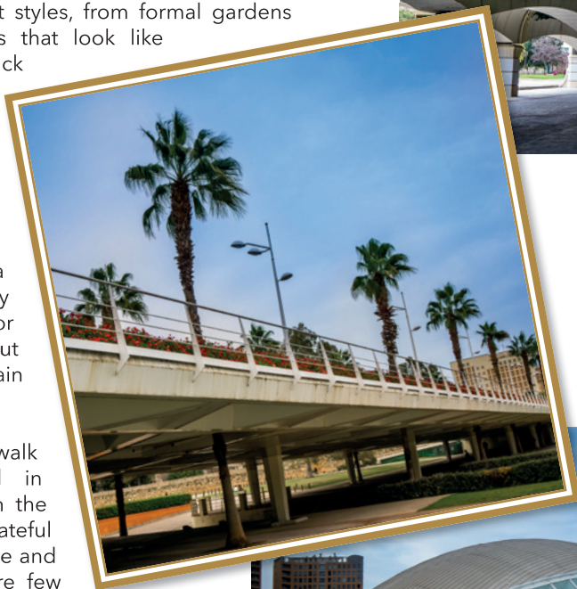
The palms grow directly through the centre of this bridge
